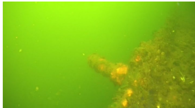
Figure 1: Remote operated vehicle photo of the submerged, protruding lag bolt.
